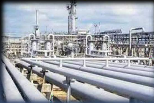
HPCL Pipeline work
