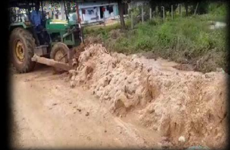
Backfilling
