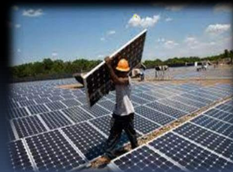
Solar panels installation
