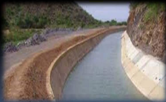
HNSS canal work
